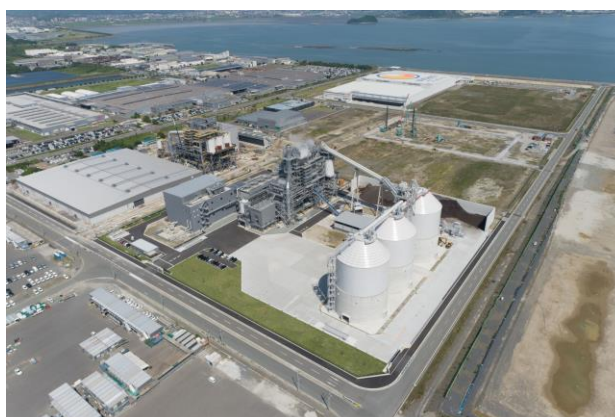
(Kanda Biomass Power Plant/photo taken in June 2021)
